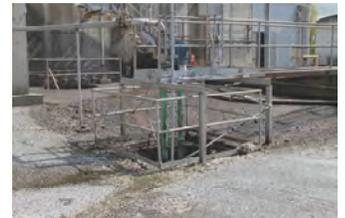
The chip pile sump collects rainwater and chips from the chip pile area. Wood chips are one of a chopper pump's favorite foods!
