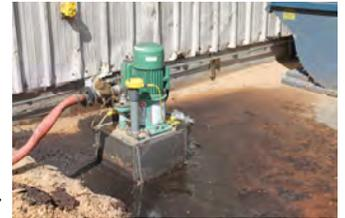
Simpson also replaced their plant sewage pump with a chopper. They almost forgot about this one too since it has not clogged in over three years.
