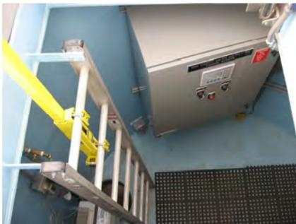
operated. The vault also includes a packaged hypo chlorination system. The first two pictures on this page show the intertie vault during transport and installation. The others show the interior components including the controls, Cla-Val's and the chemical injection system.
