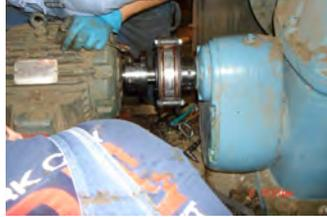
One of their large circulating pumps experienced surging due to its location in the process line. The surging resulted in coupling, seal, shaft and motor failures. After many attempts to resolve the problem they installed a MagnaDrive coupling and no failures have occurred.
