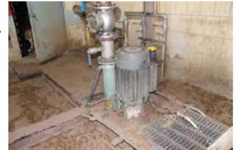
The bug pit collects process water from the clarifiers and uses a vertical Vaughan chopper to replace a non-clog that also clogged continuously. The chopper has not clogged in the three years since it was installed. In fact, they almost forgot it was there!
