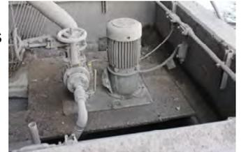
Another is the stock chest sump. The pump in this sump recirculates the paper stock which has a consistency similar to that of oatmeal. This pump clogged continuously and since it was replaced with a Vaughan chopper there have been no clogs.
