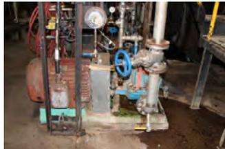
The photo to the right is the gear drive that powers the ash conveyor. A magnetic coupling provides a cushioned start that protects the motor when the belt is jammed or plugged.
