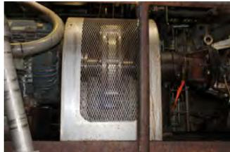
A split case pump that provides lubricating water to the mechanical seals of two digesters was tripping its breaker due to high amps. The standard option would have been to install a larger motor but, the retrofit would have been difficult and the downtime was unacceptable. The MagnaDrive coupling was gapped to allow a small amount of slippage which resulted in a lower FLA and thus eliminated the tripping problem.
