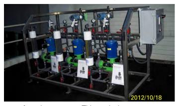
manufacturing process. This particular process required a reliable, non-metallic pump end with smooth, non-pulsing flow so Grundfos DMH dual diaphragm pumps were selected for the application. Pulsation dampeners were also incorporated to assure even smoother flow. Two pumps provide flow to two locations on the paper machine while the third
