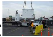
facility. The station, the largest one ever built by PumpTech, was 12ft in diameter and 34ft deep. It included three 1500 gpm Vaughan chopper pumps, a Vapex odor control system and a complete control package. This lift station has been operating flawlessly for over 5 years. The top two photos show the 421 and the associated valve vaults during unloading. The
