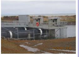
deepens the path to the ocean. They designed a pumping system incorporating 3 large vertical turbine pumps located within the reservation and beside the river near the new tribal fish hatchery.
