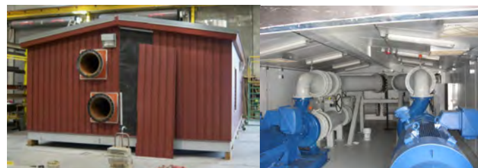
Packaged Pump House Exterior & Interior
