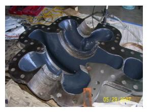
not be fully answered for many years but, a greater understanding is achieved as time goes on. MCWA tests all of the pumps every six months for performance changes that could indicate premature coating failure. They also remove the upper casings annually and inspect the coating integrity. This detailed monitoring will continue to provide the information necessary to fully answer that question.
